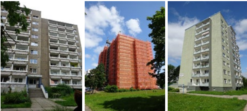
Figure 3. Nine-storey buildings in the case study area in different phases of the refurbishment process (photos by the authors).
