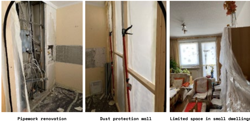
Figure 4. Renovation of apartments that were occupied (photos by the authors).
